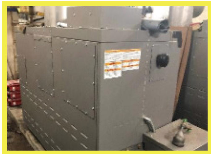
New boiler installation in progress.
